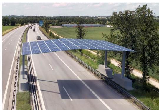
A81 Autobahn: Solar roof over the highway. Font: Austrian Institute of Technology
